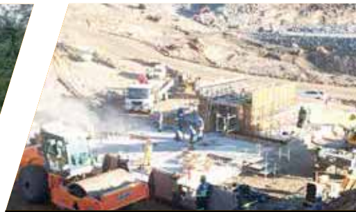
LIQHOBONG • DIAMOND MINE LESOTHO
